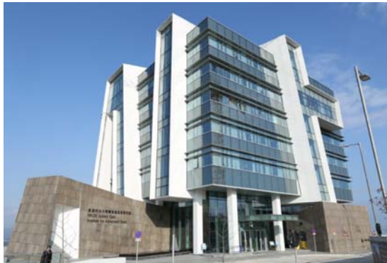
IAS Building @ HKUST
